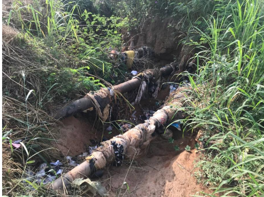
Figure 1.5: Exposed pipelines in Baruwa
